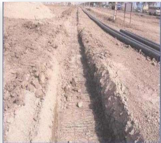
Figure-10 Excavation of polyethylene pipe trench - Site B of Arvand Free Zone (1388)
