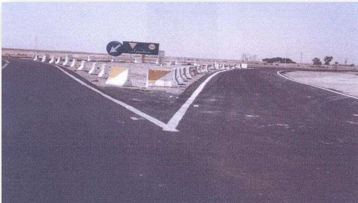
Figure-2 View of the marking and safety intersection of origin 1, located in the axis of Mahshahr - Ahvaz, Khuzestan Road and transportation (1384)
