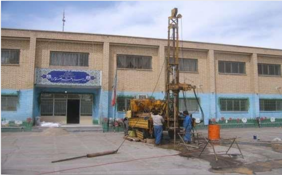
Figure-23 Machine trial borehole drilling operation of Baqerul Uloom Shahriar school, equipping Tehran schools (1388)
