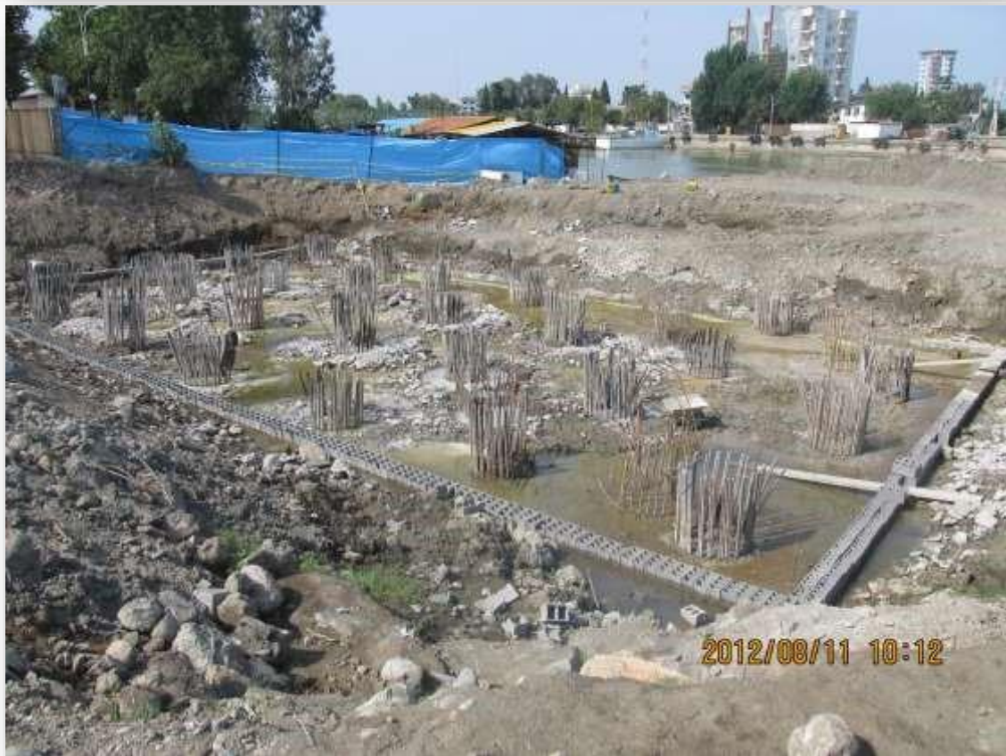
Figures- 13 & 14 Pile drilling operation of Babolsar bridge foundation (1391)
