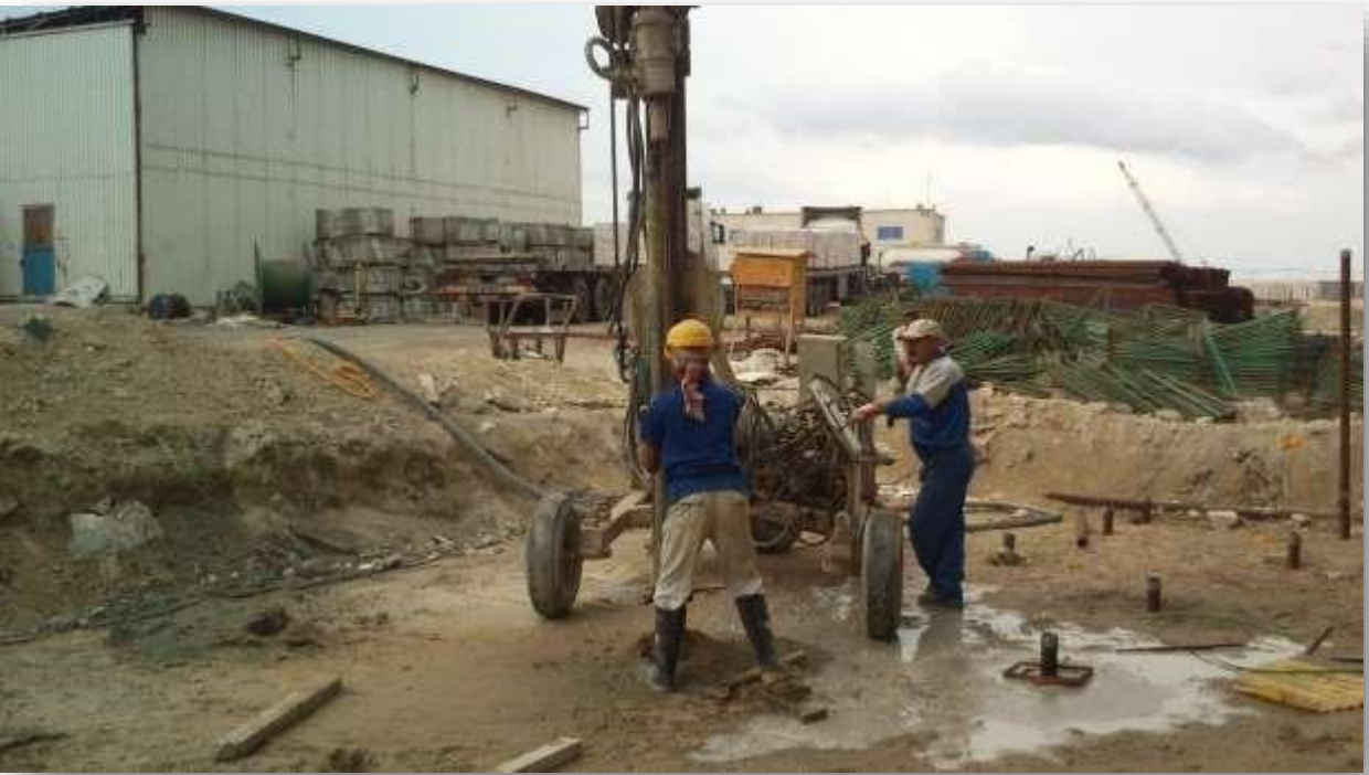
Figures-7 & 8 Micro-pile implementation operation project in Meraj Qeshm (1390-1391)
