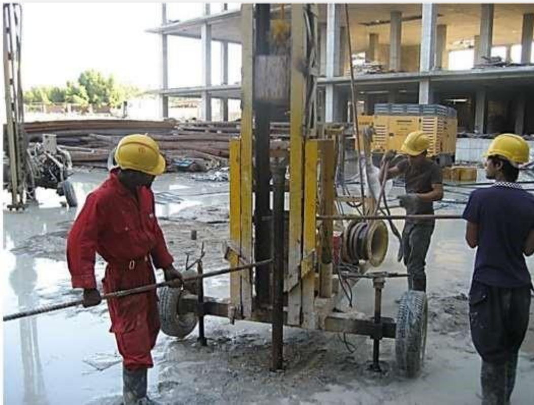
Figure-6 Micro-pile implementation operation project in Meraj Qeshm (1390)
