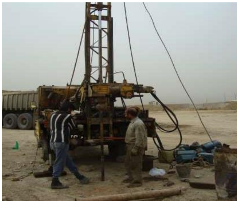
Figure-2 Drilling operations in Yaftabad residential complex, Naji Sazan Amin (1388)
