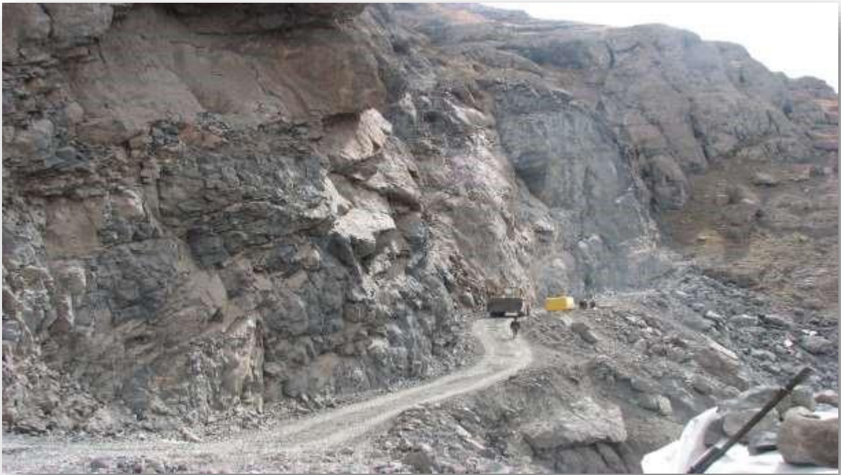
Figure-7 Mountaineering operations and preparation of potholes for explosion in station 6+200 km of Yalrud-Sorkhak
