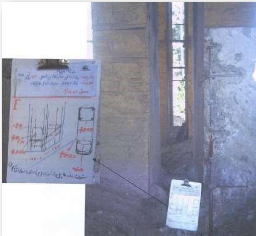
Figures-11 & 12 Sounding test of International Exhibition bridge located on Chamran Highway, Technical and Engineering Consulting Organization of Tehran city (1389)
