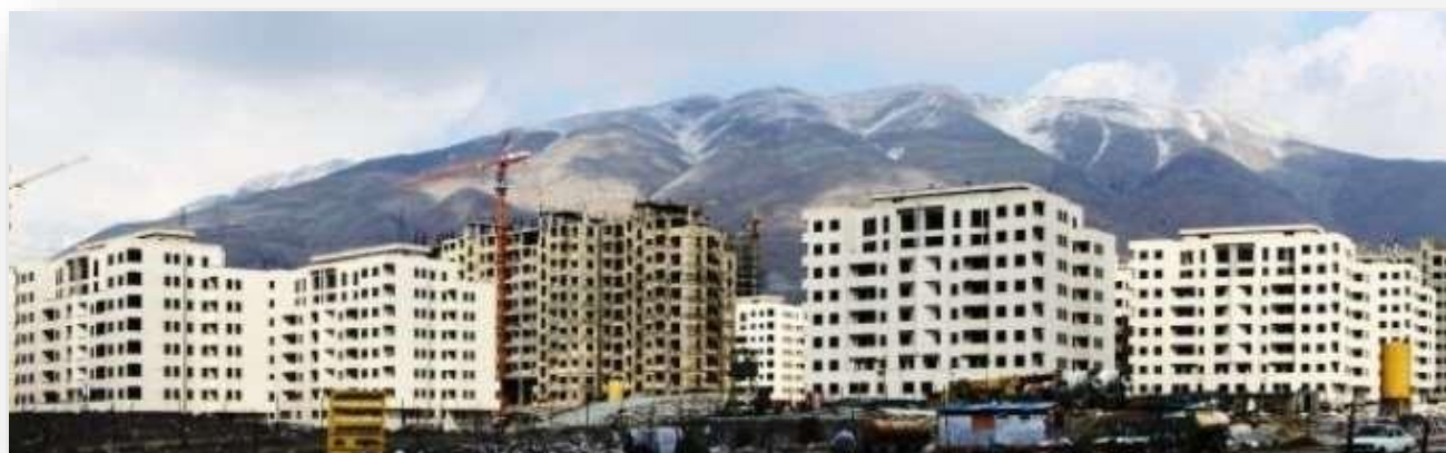
Figures-15 & 16 Views of Negin Gharb project (1391)
